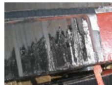
Side of a bar deeply damaged by vibration sparking
