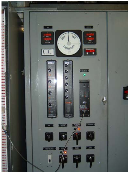
Fig. 8 Front of the New Protection and Synchronizing Control Sub-Panel Installed
